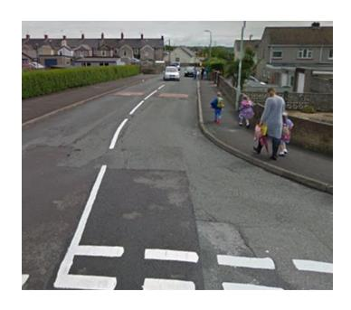
The route proceeds along Garfield Avenue and follows the continuous pavement into an un named road. Again the pavement is in good order at this point although a dedicated crossing point with dropped kerbs and tactile paving could be installed at this point to enable safe access eastwards along Garfield Avenue and onwards to Litchard Hill.
