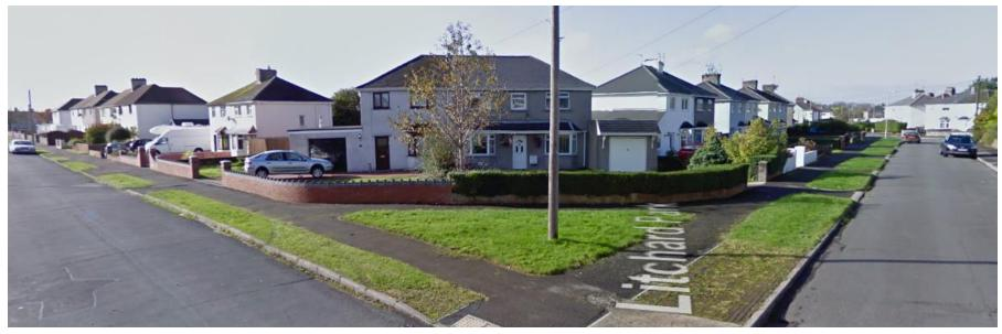
The pavement along |Litchard Park as it progresses along Route 2 towards Pendre is in good order and suitable for incorporation into the active travel route. Although as Litchard Park heads eastwards towards Coity Road the tactile paving is inadequate and will need to be upgraded.
